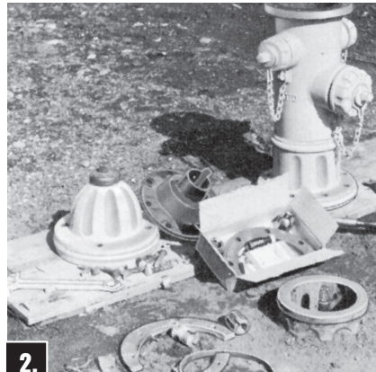
2. Unbolt and remove broken Traffic Flange from Upper Barrel. Remove Weather Cap, Hold Down Nut, and Operating Nut from Bonnet. Lubricate Brass Sleeve and slide over threaded Stem end to prevent O-ring damage. Unbolt Bonnet from Upper Barrel. Slide Upper Stem out of Bonnet. Remove damaged Stem Coupling and Sleeve from Upper and Lower Stem.
