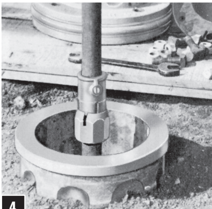
4. Turn Stem Coupling and Upper Stem so that slot in Thimble aligns with the tongue and groove of Stems. Hold Upper Stem in alignment and screw Stem Coupling upward until tongue and groove of Stems firmly lock together. Tighten with wrench. With Stem Coupling in place, slide Sleeve downward so that lower end of Sleeve surrounds upper end of Stem Coupling. Be sure Sleeve projections fit into Stem Coupling slots. With Sleeve in place, tighten set screw in Sleeve.
