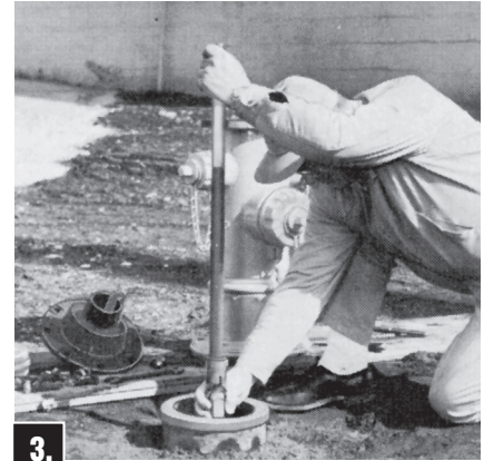
3. Place new Stem Coupling sleeve part onto Upper Stem. NOTE: If Upper Stem of Hydrant is 1 1/4" In diameter, cut sleeve as Indicated by lettering on sleeve. Screw new Stem Coupling part onto Lower Stem as far as threads permit. Screw Upper Stem into Stem Coupling until it contacts the Lower Stem.
