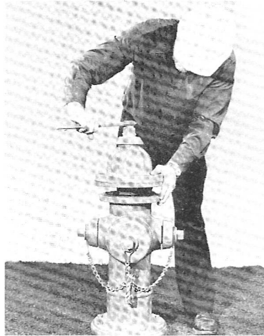
2. Turn operating nut in opening direction while holding bonnet stationary until stop nut bottoms. This lifts bonnet off upper barrel.
