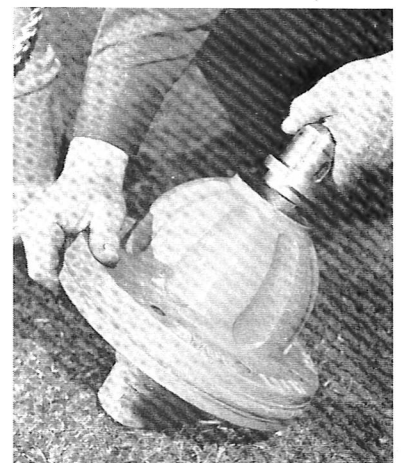
6. Remove operating nut, stop nut assembly and thrust washer by lifting out of bonnet. Remove hold down nut by turning it in hydrant closing direction.
