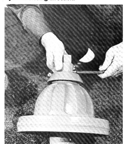
9. Attach weather cap and lock in place by tightening set screw. IMPORTANT - Now turn operating nut in opening direction until stop nut "bottoms out" (full open position).
