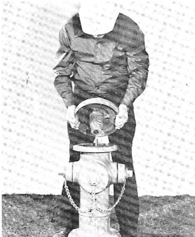
4. Lift bonnet from Hydrant. Other operations may now be performed on the hydrant.
