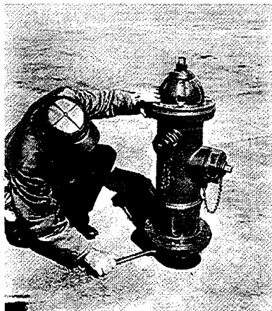
1. Loosen nuts on safety flange bolts.
