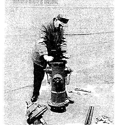
11. Rotate guide plate assembly clockwise until contact is made with upper barrel flange. Continue to rotate guide plate clockwise to raise center portion of wrench and stem assembly to close main valve of hydrant. CAUTION: Only rotate guide plate until main valve is moved to closed position since seat ring only has small contact with shoe bushing at this time.
