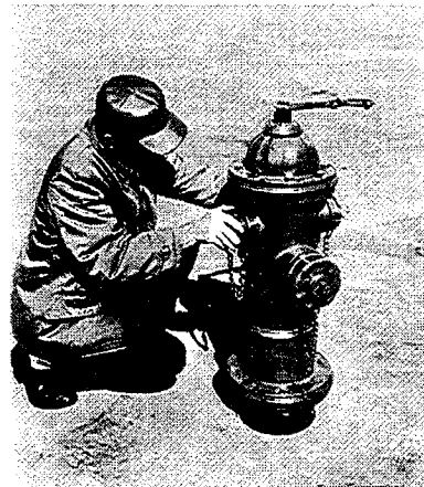
3. Rotate upper barrel section as desired.
