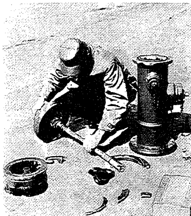
4. Remove upper stem from stem nut by holding bonnet and turning stem counter-clockwise.
