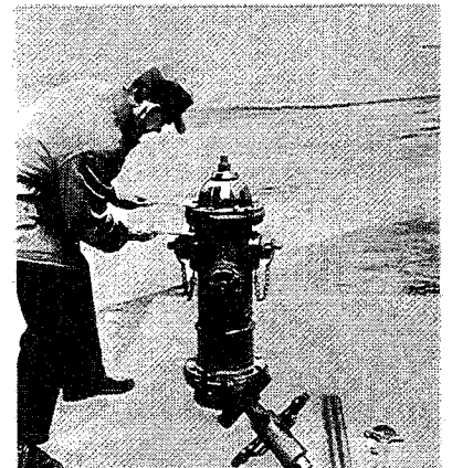
15. Rotate operating nut in closing direction which lowers bonnet assembly onto upper barrel and allows bolts to be replaced. With all bolts in bonnet, rotate operating nut using the same torque as normally used to close the hydrant. Tighten all bonnet bolts and nuts. Loosen one hose nozzle cap, to bleed air, while hydrant is opened to check gasket tightness. When barrel is filled with water, tighten nozzle cap and check gaskets. Turn operating nut and weather cap to fully closed position. Loosen one nozzle cap to allow barrel to drain.
