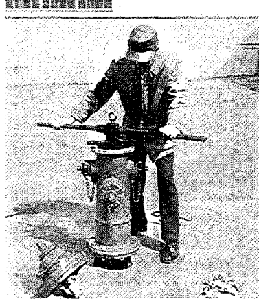
10. Slowly lower entire wrench and stem assembly into hydrant barrel until seat ring threads engage shoe bushing. Rotate seat wrench clockwise approximately 2 revolutions to start seat ring into shoe bushing.
