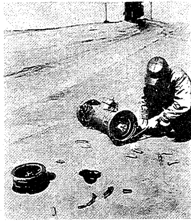
2. Unbolt and remove broken safety flange from upper barrel.
