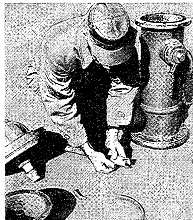
5. Remove stainless steel cotter pin from stainless steel clevis pin. Remove stainless steel clevis pin and remove safety stem coupling from upper stem.
