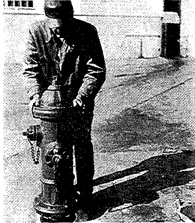
11. Check bonnet gasket on top of upper barrel, replace if damaged. Check to see that upper stem threads are lubricated and upper stem seal ("O" Ring) is not damaged. Rotate the operating nut in opening direction to fully open position. This extends stem nut. Reassemble bonnet assembly to upper stem by rotating clockwise as far as possible, then back up only enough to align bolt holes, if needed.
