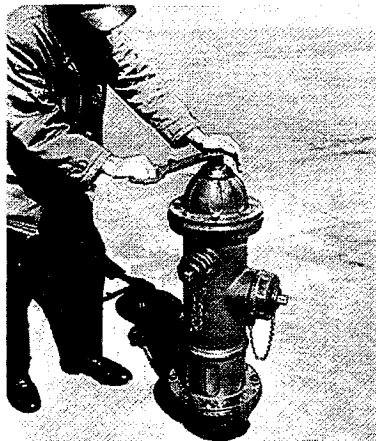
2. Turn operating nut slightly in the opening direction to relieve compression between barrel sections.
