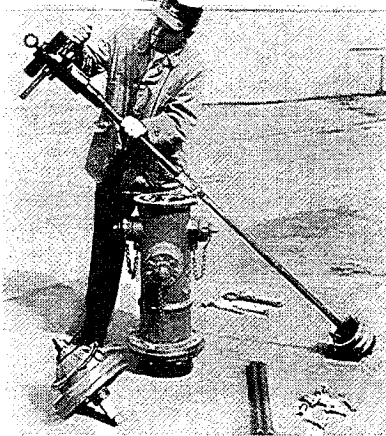
9. Retract guide plate on seat wrench to uppermost position by rotating counterclockwise.
