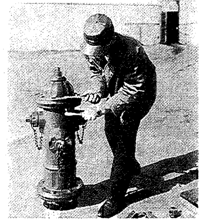
12. Rotate operating nut in closing direction which lowers bonnet assembly onto upper barrel and allows bolts to be replaced. With all bolts in bonnet, rotate operating nut using the same torque as normally used to close the hydrant. Tighten all bonnet bolts and nuts.
