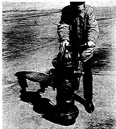
4. Tighten operating nut, turning in closing direction.
