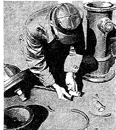
6. Assemble new safety stem coupling to upper stem with new stainless steel clevis pin and new stainless steel cotter pin.
