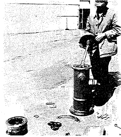
3. Unbolt and remove bonnet and upper stem from upper barrel.
