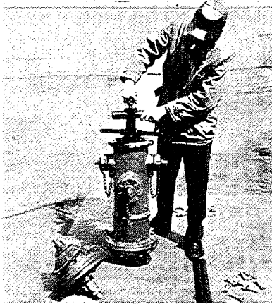
13. Remove bonnet bolts from guide plate holes and rotate clockwise to bring stem and main valve to fully closed position. Open control valve ahead of hydrant to reapply line pressure. Detach seat wrench from stem by turning eyebolt counterclockwise until threads disengage and then lift complete wrench off stem.
