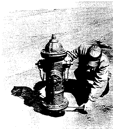
5. Tighten safety flange bolts.
