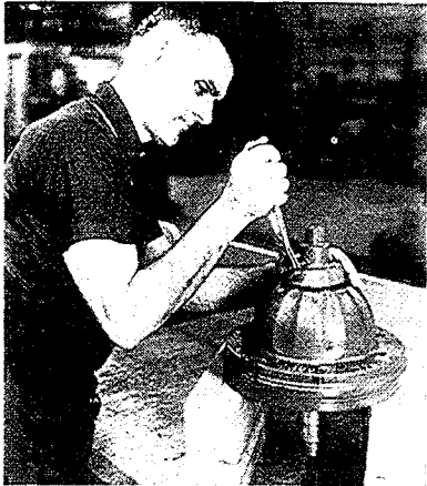
1. Remove socket head screw pin from combined operating nut and weather cap.
