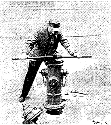
9. Retract guide plate on seat wrench to uppermost position by rotating counterclockwise.
