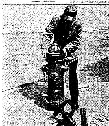
14. Replace bonnet gasket on top of upper barrel and see that upper stem threads and upper stem seal ("O" Ring) are thoroughly lubricated with a light cup grease. Check to be sure that the operating nut is in the fully open position which is with the stem nut fully extended. Reassemble bonnet assembly to upper stem by rotating clockwise as far as possible, then back up only enough to align bolt holes, if needed.
