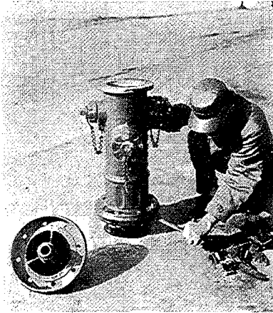
10. Check safety flange gasket on lower barrel and if damaged, replace. Reassemble upper barrel being sure gasket is centered as nozzles are located in desired position. Bolt into place the two halves of safety flange with circular groove facing upward, and with safety flange fitting snugly around lower barrel.
