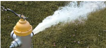
STEP 2: INDUCE NOISE INTO THE PIPE
