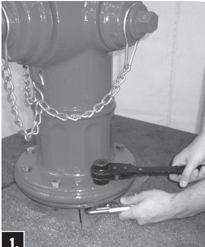
1. Loosen Nuts on Traffic Flange Bolts.
