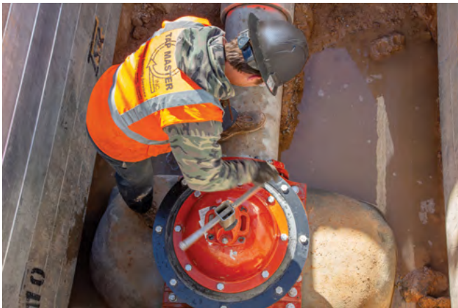
FIGURE 3 - THE PERMASEAL INSERTION VALVE FULLY INSTALLED FOR THE CITY OF PHOENIX WATER SERVICE DEPARTMENT.
