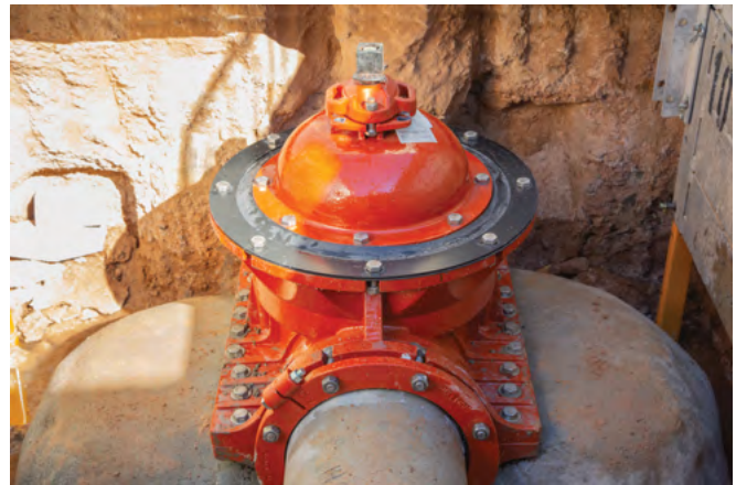
FIGURE 3 - THE PERMASEAL INSERTION VALVE FULLY INSTALLED FOR THE CITY OF PHOENIX WATER SERVICE DEPARTMENT.
